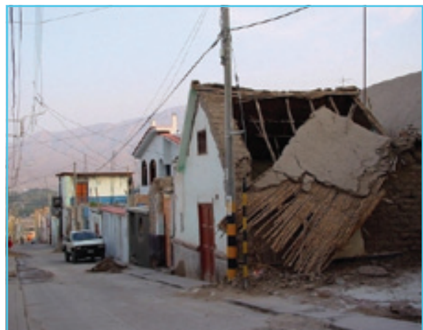
The inhabitants of this house in Moquegua, Peru had a narrow escape, because the failing roof slid sideways rather than falling in on them.
