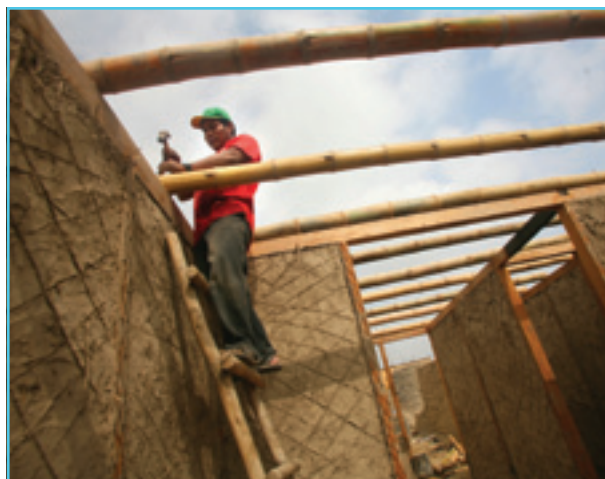
Improved quincha , used here in reconstruction after an earthquake in Chinchá, Peru, is proven to have good earthquake resistance.
