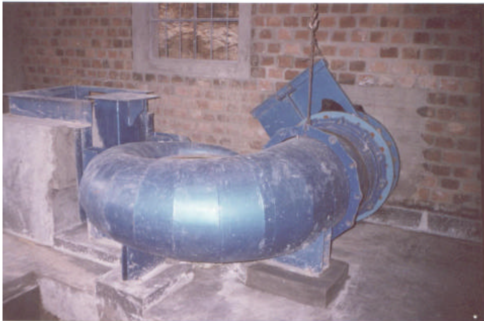
Fig. 1 and 2 Leveling and Anchoring of the Axial Turbine Frame.
